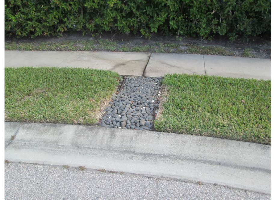
Remove existing gravel and install 8" x 4" sidewalk flume on Valenza Ct
