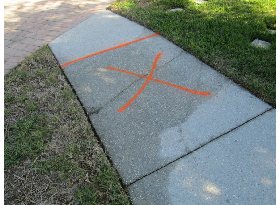
Remove and replace 6' x 5' panel on Savona Way cul-de-sac
