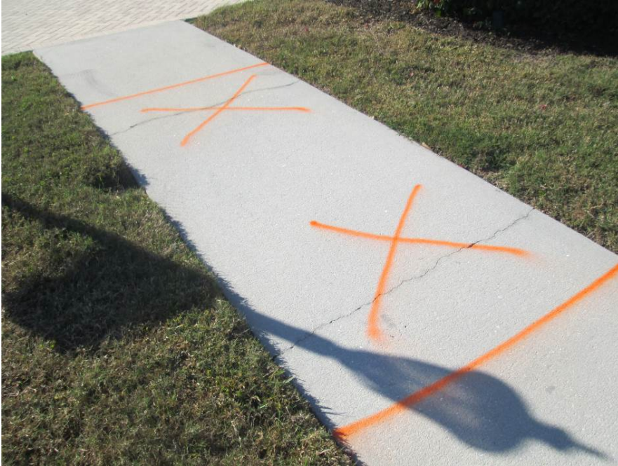
Remove and replace 5' x 5' panels on Treviso Ct west of Veneto Blvd
