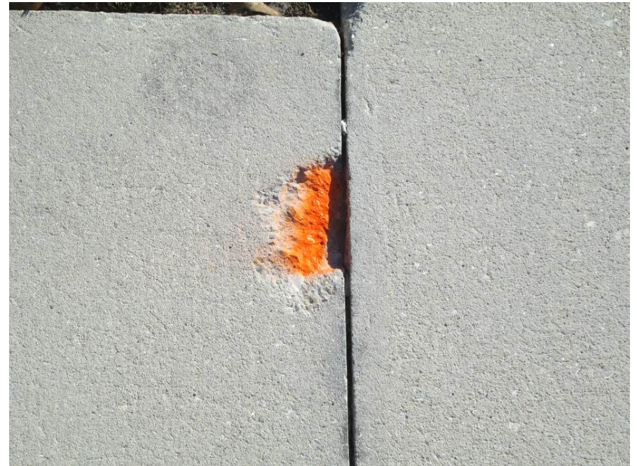
Epoxy grout sidewalk gouge on Bolanza Ct
