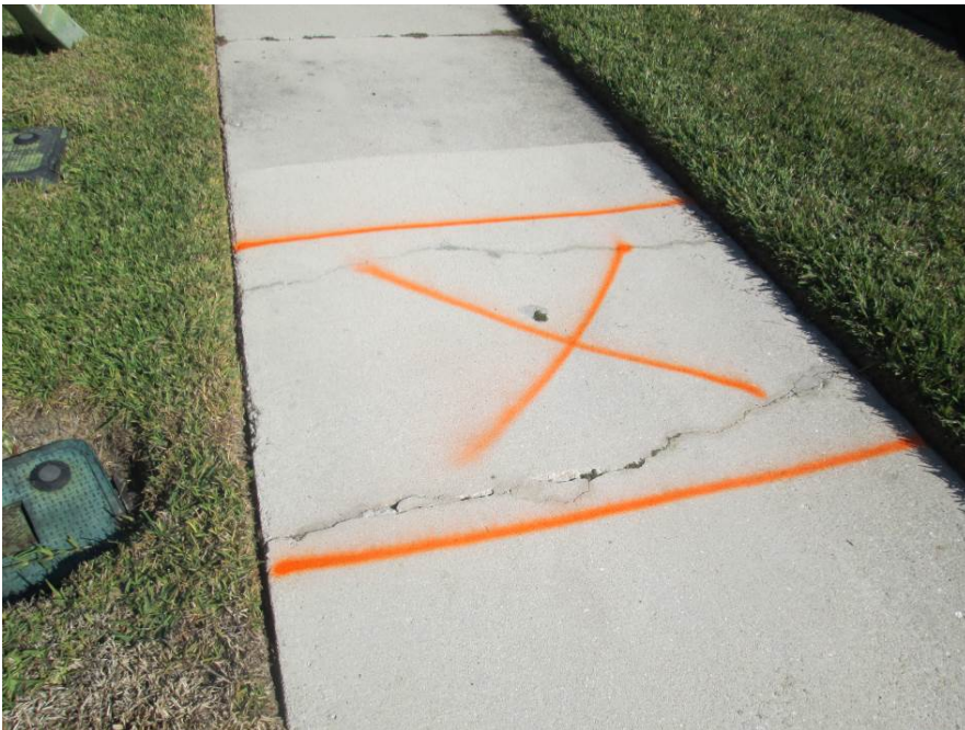
Remove and replace 4.5' x 5' panel on Padova Way east of Tiziano Way
