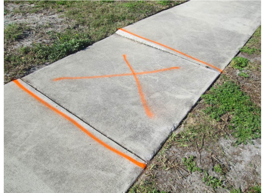
Remove and replace 5.5' x 5' panel on Padova Way south of Sevilla Pl
