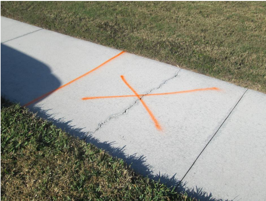
Remove and replace 5' x 5' panel on Bolanza Ct at Treviso Ct
