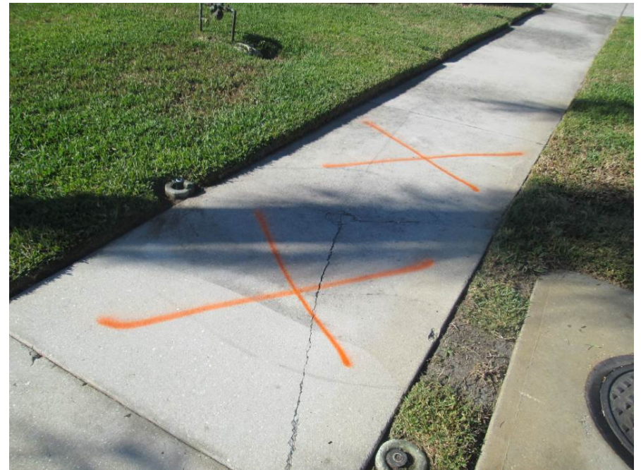
Remove and replace 11' x 5' panel on Medici Terrace
