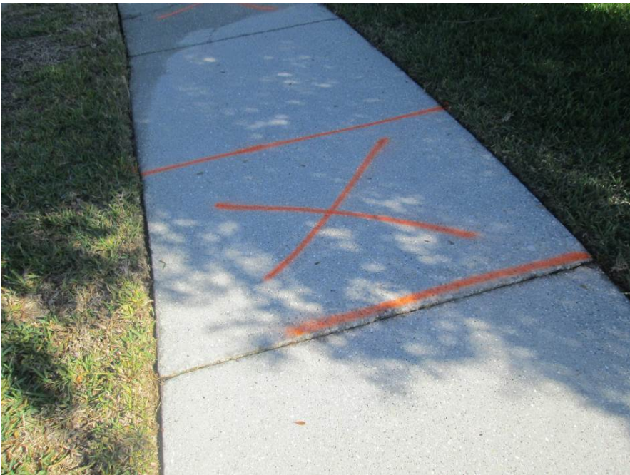
Remove and replace 5' x 5' panel on Savona Way cul-de-sac
