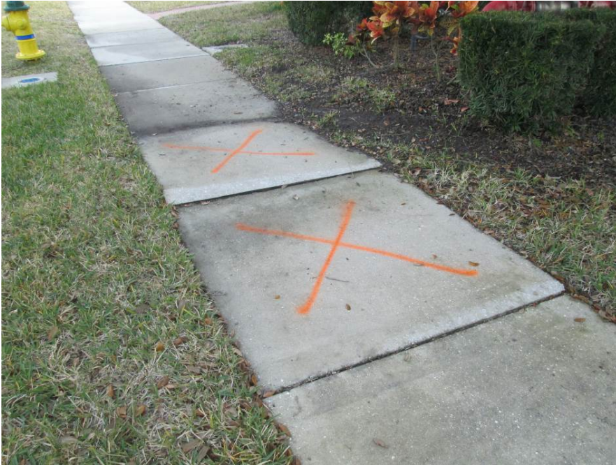
Remove and replace 5' x 5' panels on Bella Vista near tennis courts
