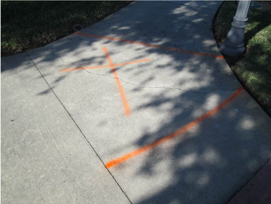
Remove and replace +/- 6' x 5' panel on SW corner of Pesaro & Terra Bella
