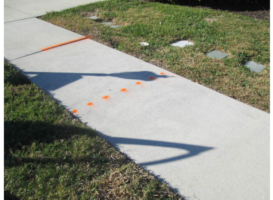
Saw cut existing sidewalk on Bolanza Ct & grind edge
