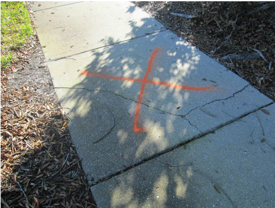
Remove and replace 5' x 5' panel on Pesaro Dr near commercial area
