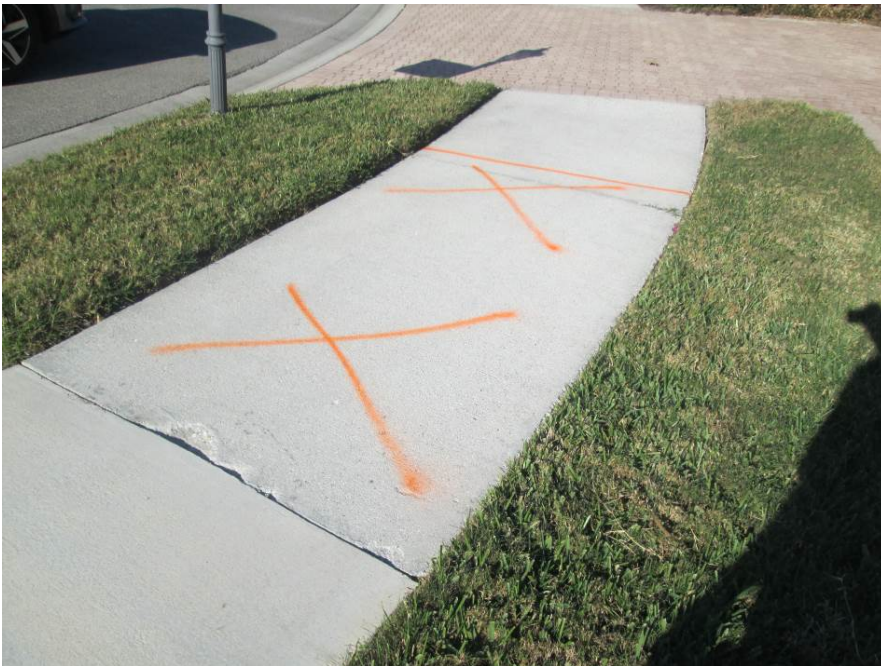
Remove and replace 9' x 5' sidewalk in Treviso Ct cul-de-sac
