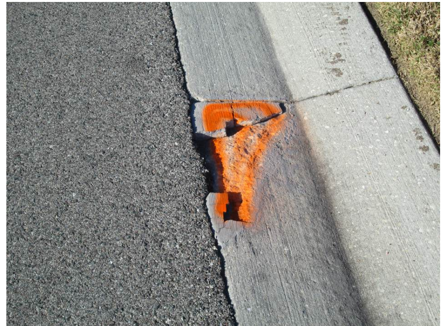
Epoxy grout damaged curb on Treviso Ct near cul-de-sac
