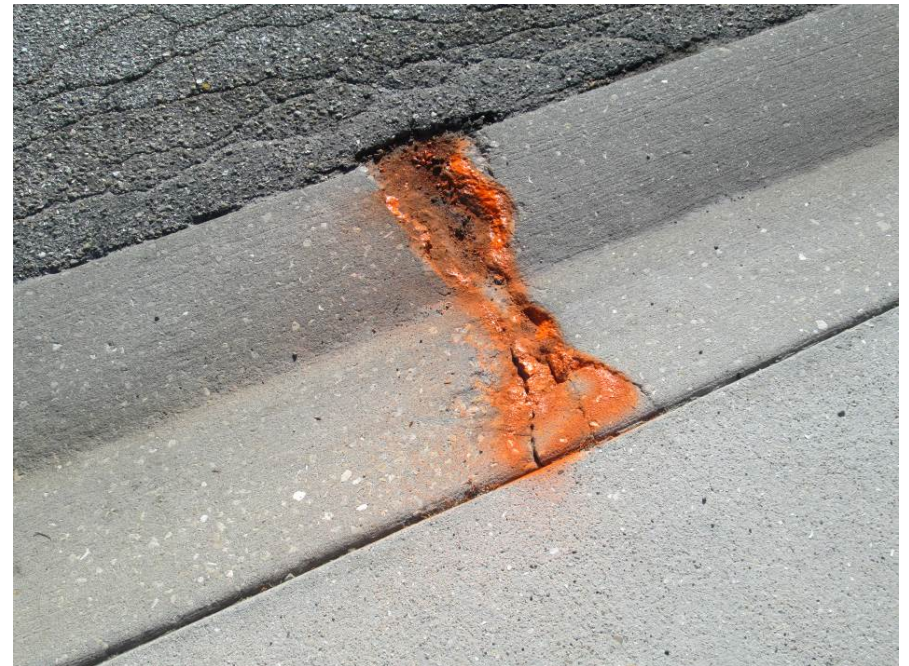
Epoxy repair damaged curb at 154 Padova Way
