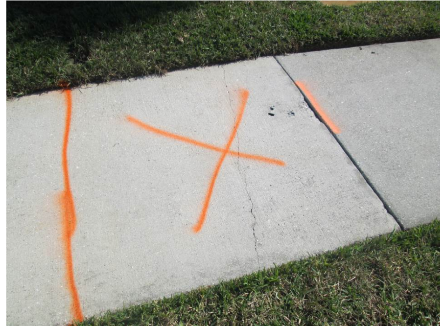
Remove and replace 5' x 5' panel on Rimini Way near east Montelluna
