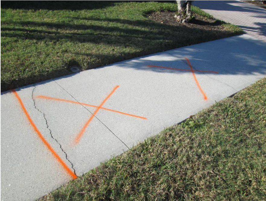
Remove and replace 5' x 5' panels on Treviso Ct south of Bolanza Ct
