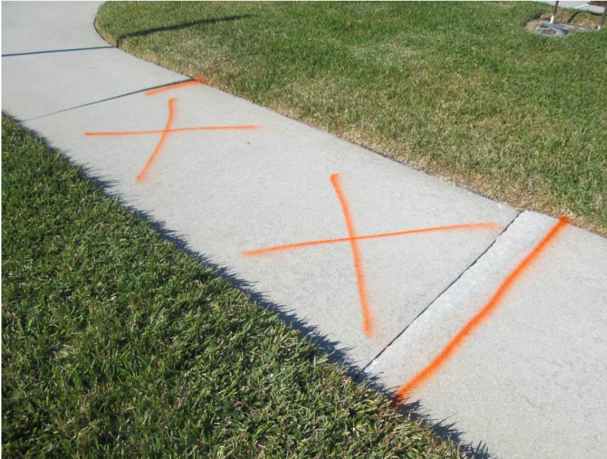
Remove and replace 5' x 5' panels on Padova Way at Montelluna
