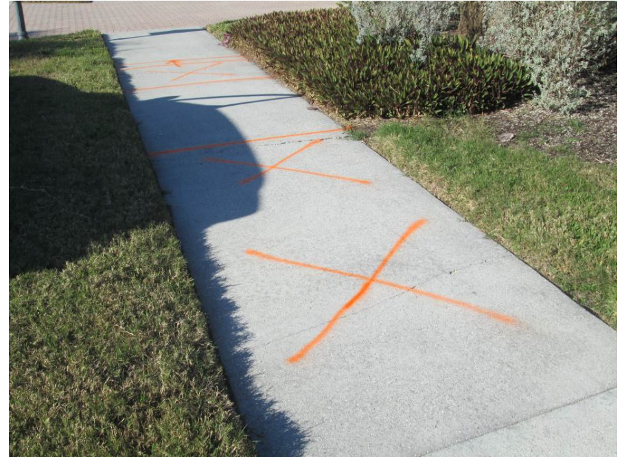
Remove and replace 5' x 5' panels on Treviso Ct near cul-de-sac
