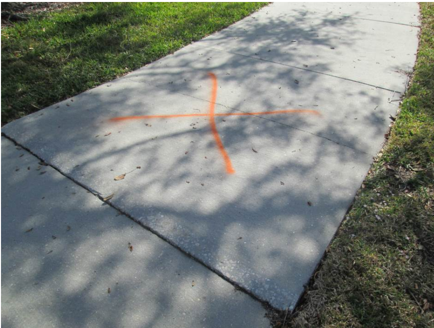
Remove and replace 9' x 8' panel on Veneto Blvd south of Padova Way
